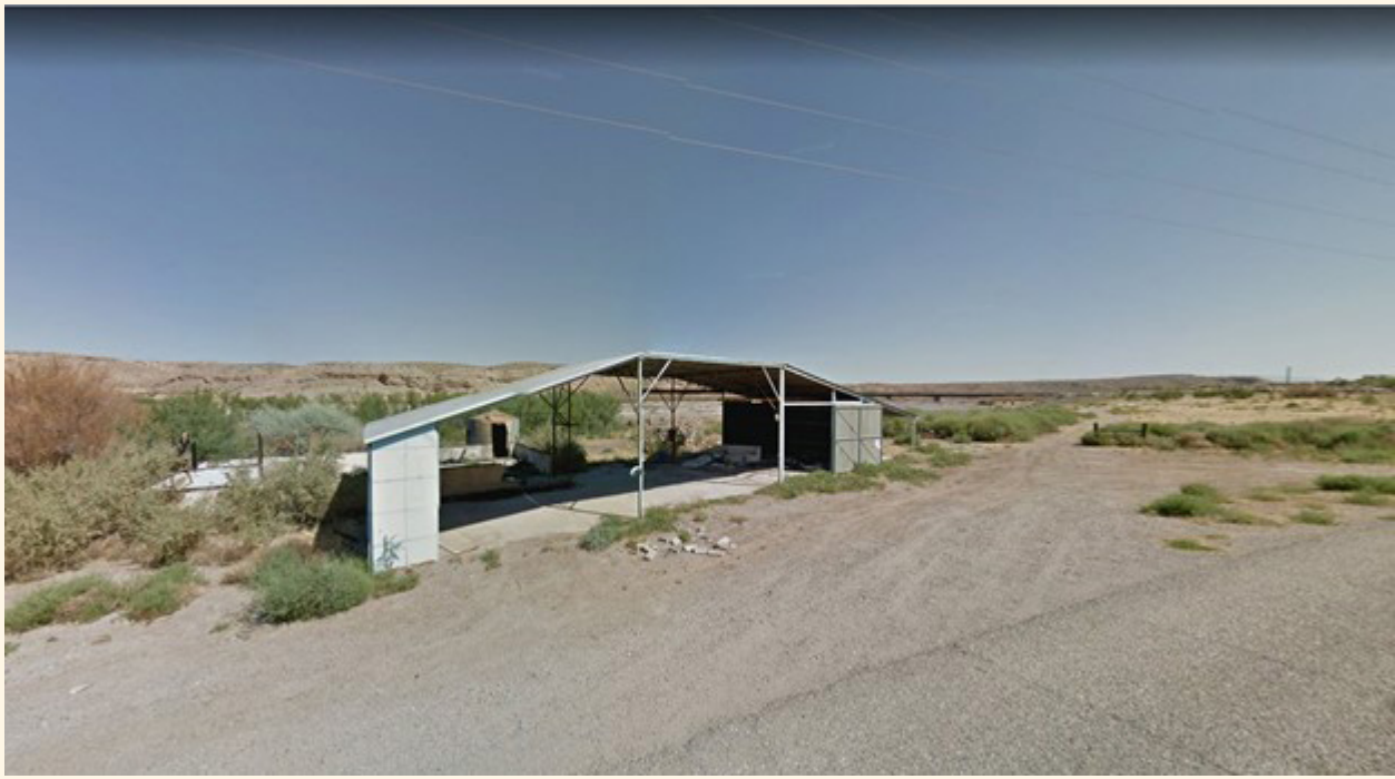
Riverside structure demo, pre
