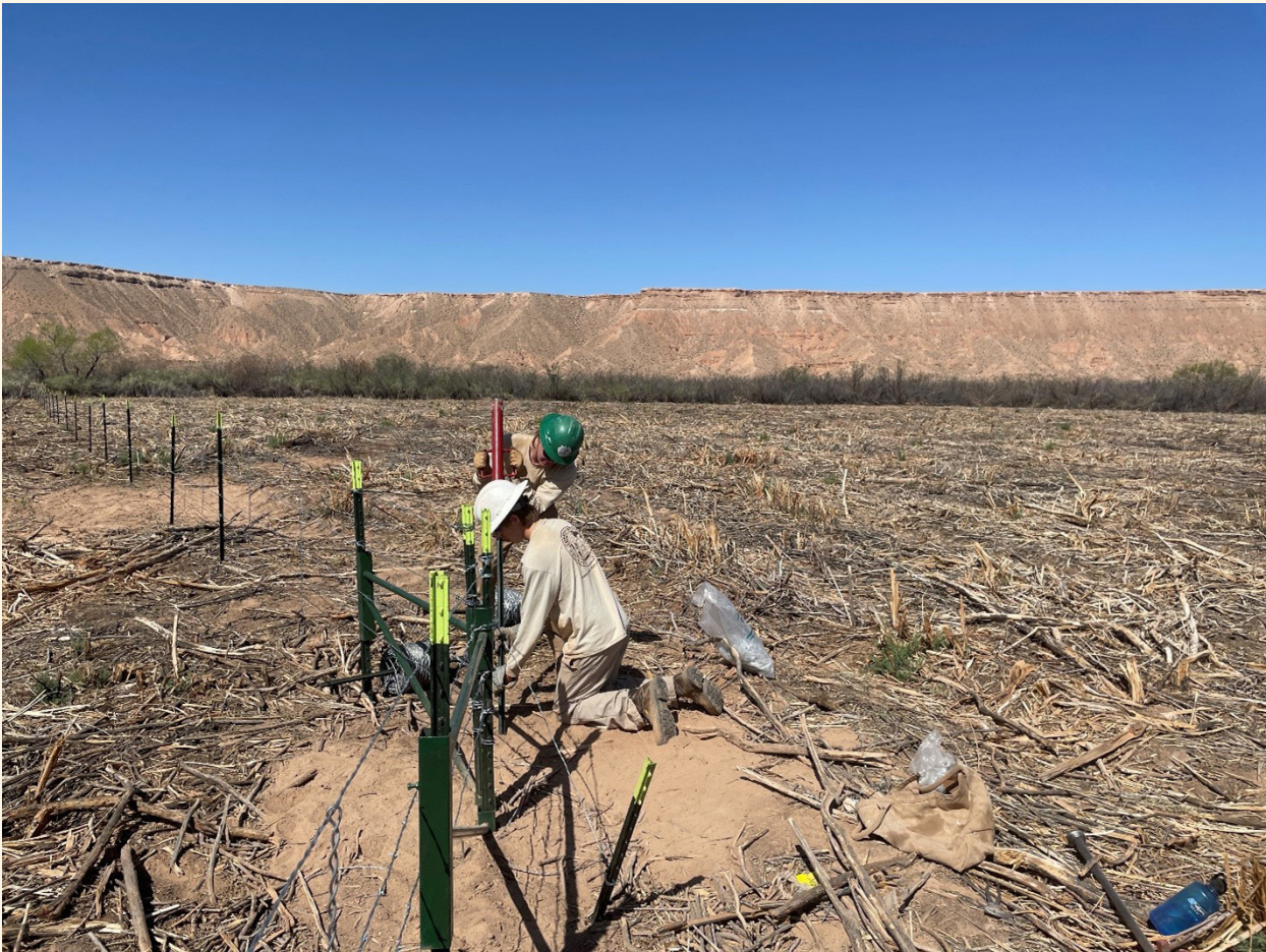
American Conservation Experience crew installing fence
