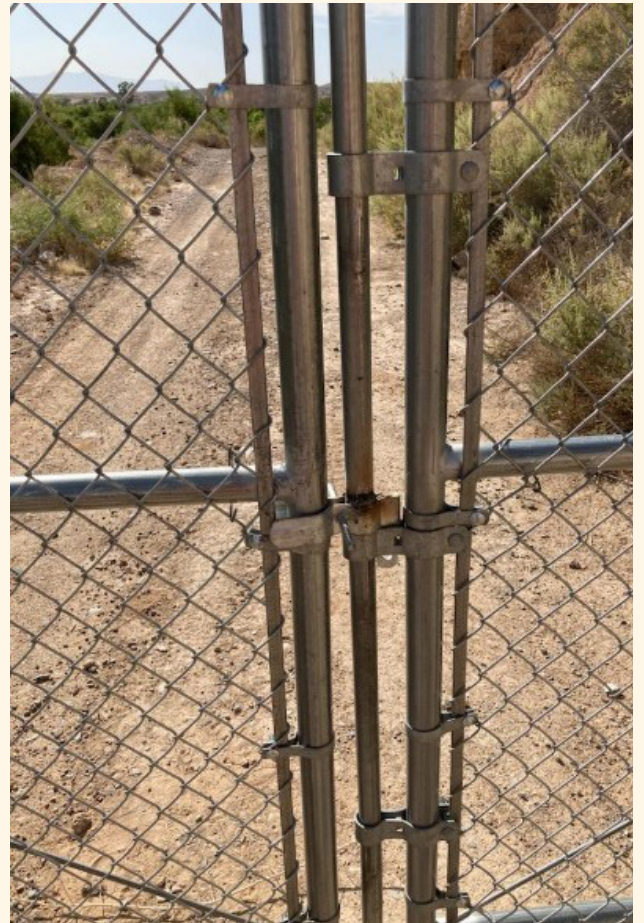
Muddy River gate repair
